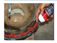
FLEXMASTER UV - UV Resistant Adhesant (Adhesive and Sealant in one)
